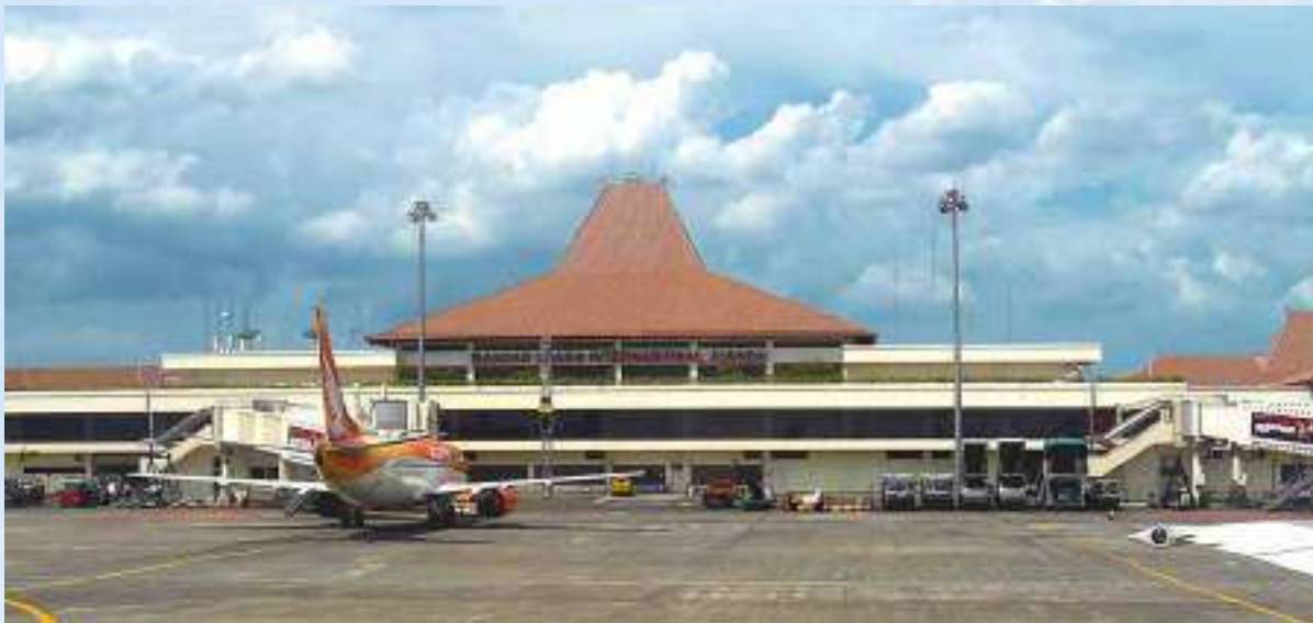
Juanda International Airport - Surabaya 5 x 1740 KVA, 4 x 2030 KVA
