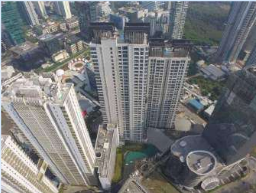
The Elements Apartment Lot 16 - Kuningan, Jakarta 2 x 2015 KVA
