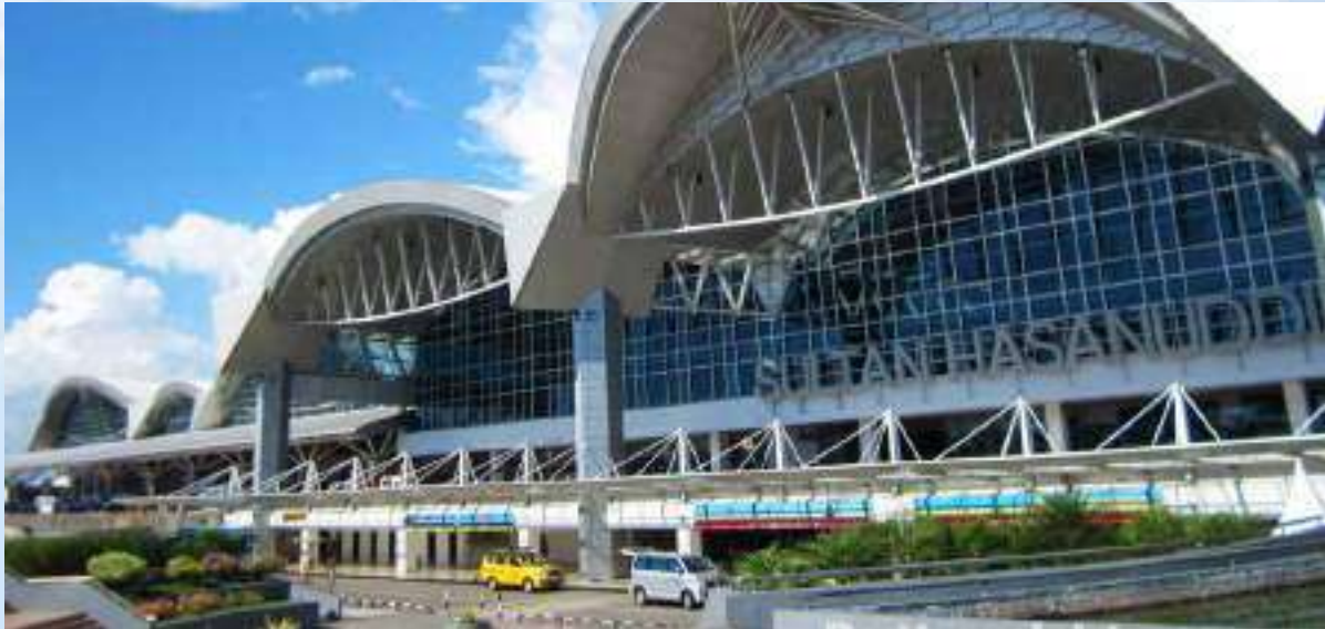
Sultan Hasanuddin International Airport - Makassar 2 X 2000 KVA, 1 X 680 KVA
