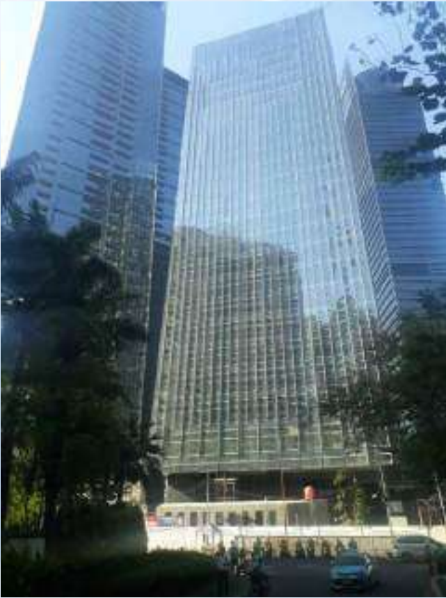
Sudirman Office 7.8, Jakarta 3 x 2015 KVA
