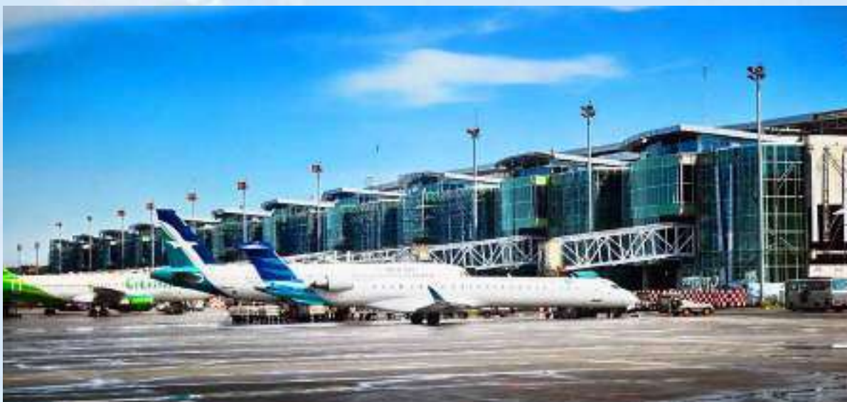
Sepinggan International Airport - Balikpapan 5 X 2030 KVA
