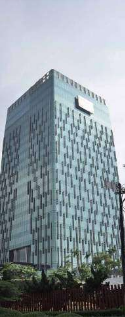
Gudang Garam Tower 2 x 2030 KVA, 1 x 1800 KVA
