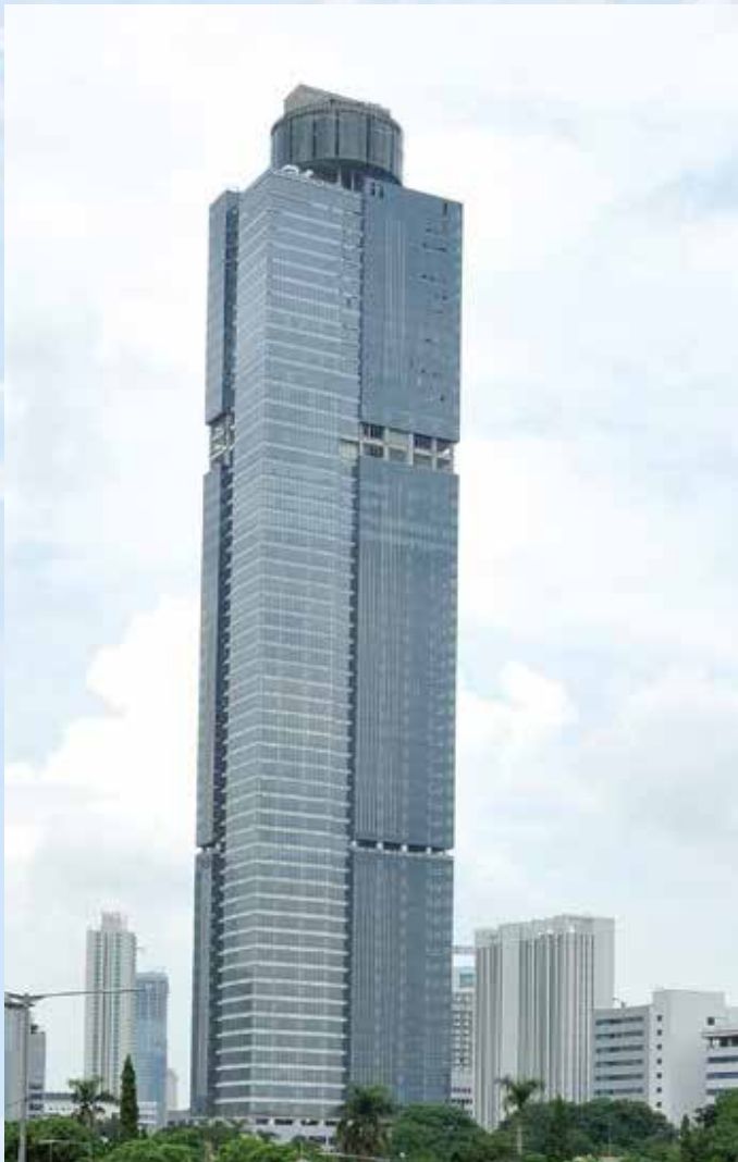
Gama Tower, Jakarta 6 x 2015 KVA
