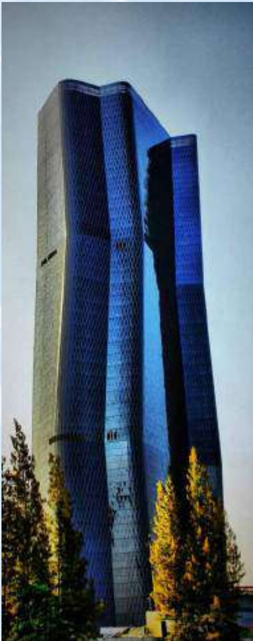
Bakrie Tower Rasuna Epicentrum 9 X 1920 KVA
