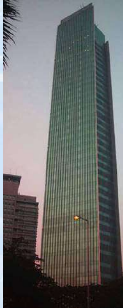
The Energy Building 4 X 2000 KVA
