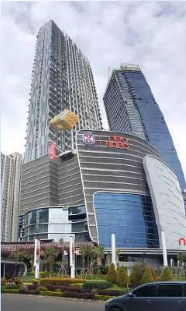
SOHO @ Podomoro City, Jakarta 3 x 1800 KVA, 7 x 2030 KVA
