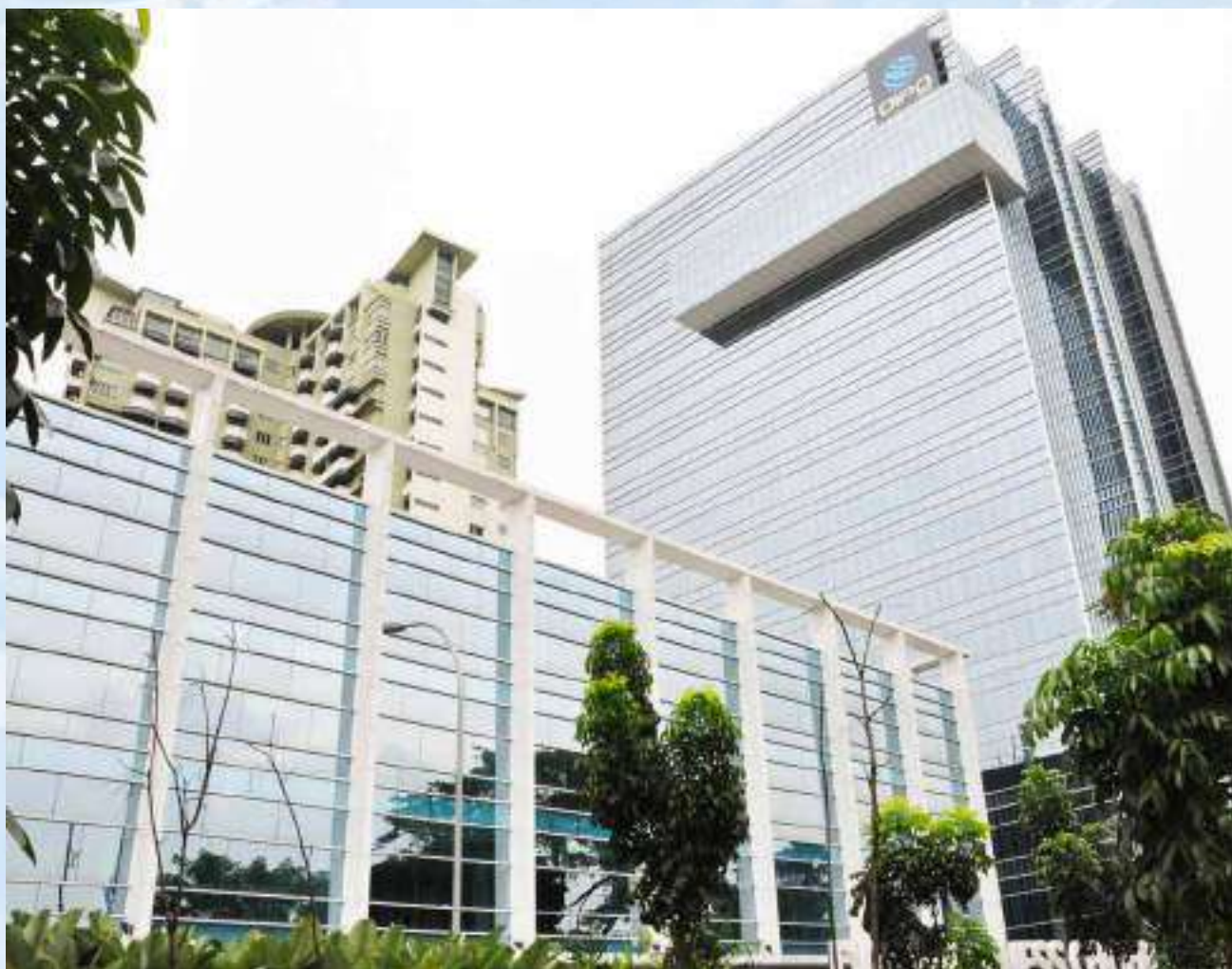
Dipo Business Center 2 X 1362.5 KVA
