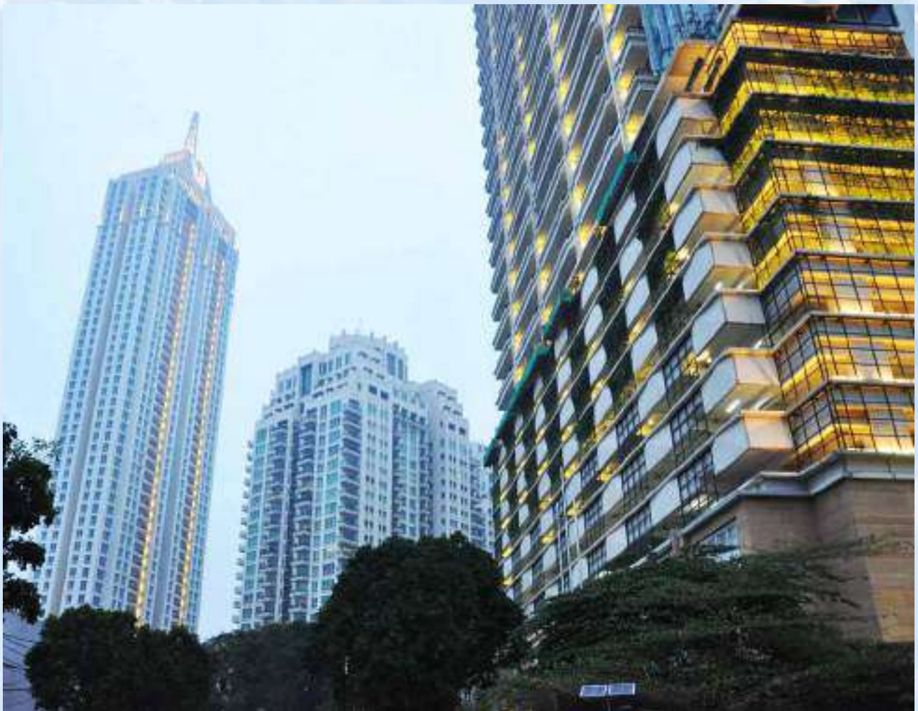
The Pakuwono Signature - 3 X 1362.5 KVA The Pakuwono House - 2 X 1450 KVA
